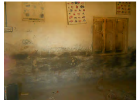
Moak Sharif Primary School, Classroom - Before
