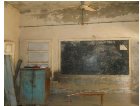
Moak Sharif Primary School, Classroom - Before
