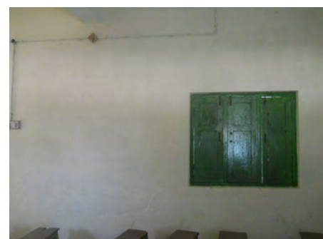
Moak Sharif Primary School, Classroom - After
