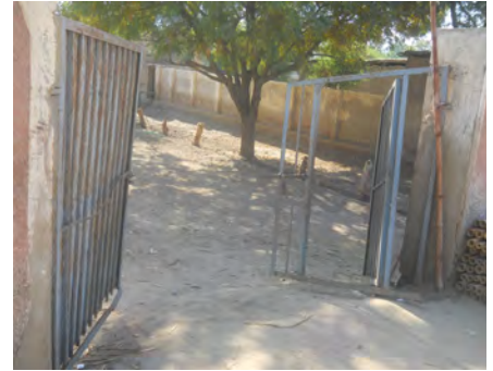
Moak Sharif Primary School, Main Gate - Before
