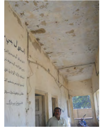
Moak Sharif Primary School Veranda - Before
